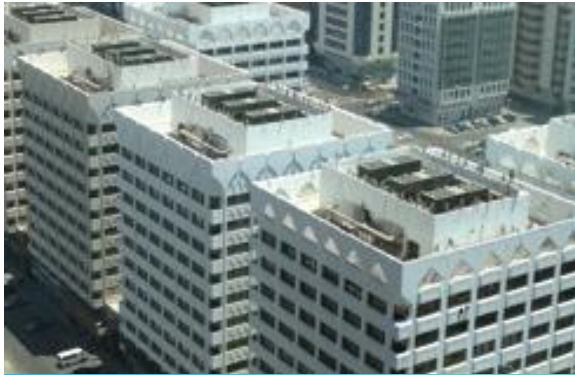
Roof Top Chillers
