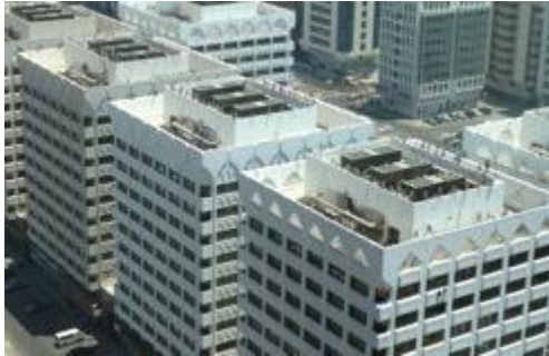
Roof Top Chillers
