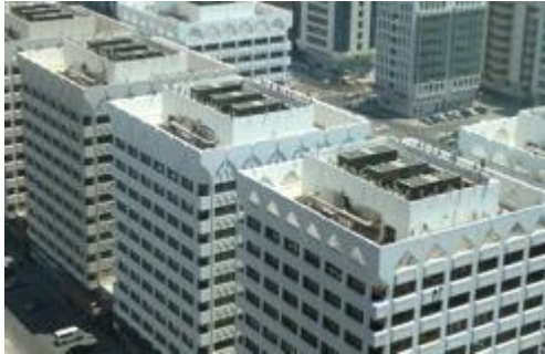
Roof Top Chillers
